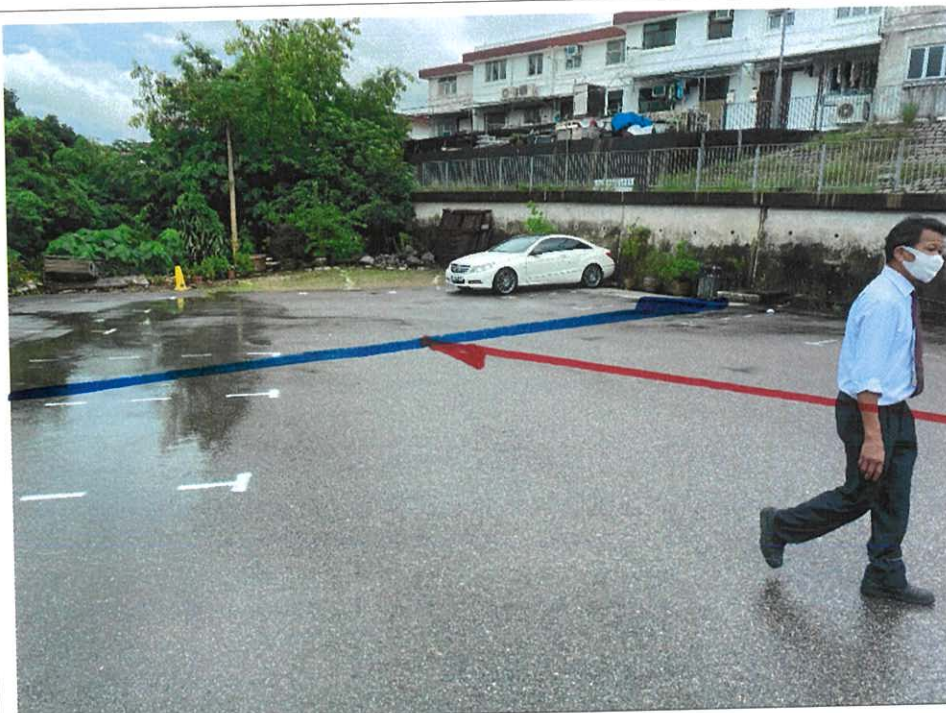
P2; shows the proposed 300 mm U-C intercepts the surface runoff from the parking area of the manhole
