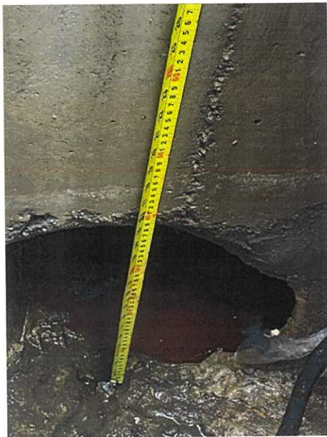
P4: Shows the approx. dimension of concrete pipe,
