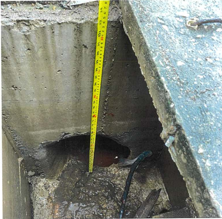
P3: shows the concrete pipe discharge
